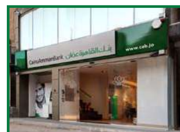
Jerash Branch Al-Qayrawan Roundabout
